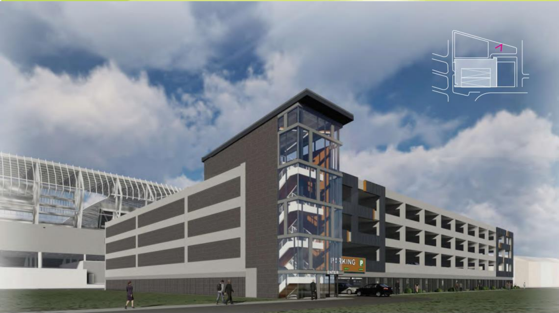
View of North Stair Looking SW North Garage
