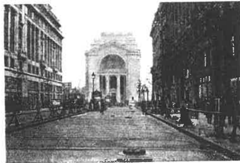
KINGSWAY, LONDON, NEW MAIN ARTERY Widening entirely paid for by "excess condemnation"
