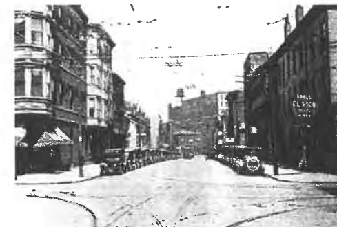
FIFTH STREET, EAST OF BROADWAY Eventually must be widened, and extended to the east over Eggleston Avenue to Third Street
