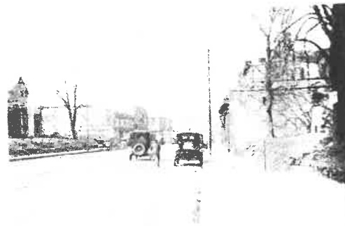
MAIN STREET, EAST ORANGE, N. J. The roadway recently widened from 40 feet to 52 feet, despite the fact that the street is only 66 feet wide, as shown, and the cost assessed locally. The property owners have since petitioned that the street itself be widened to 80 feet or more.
