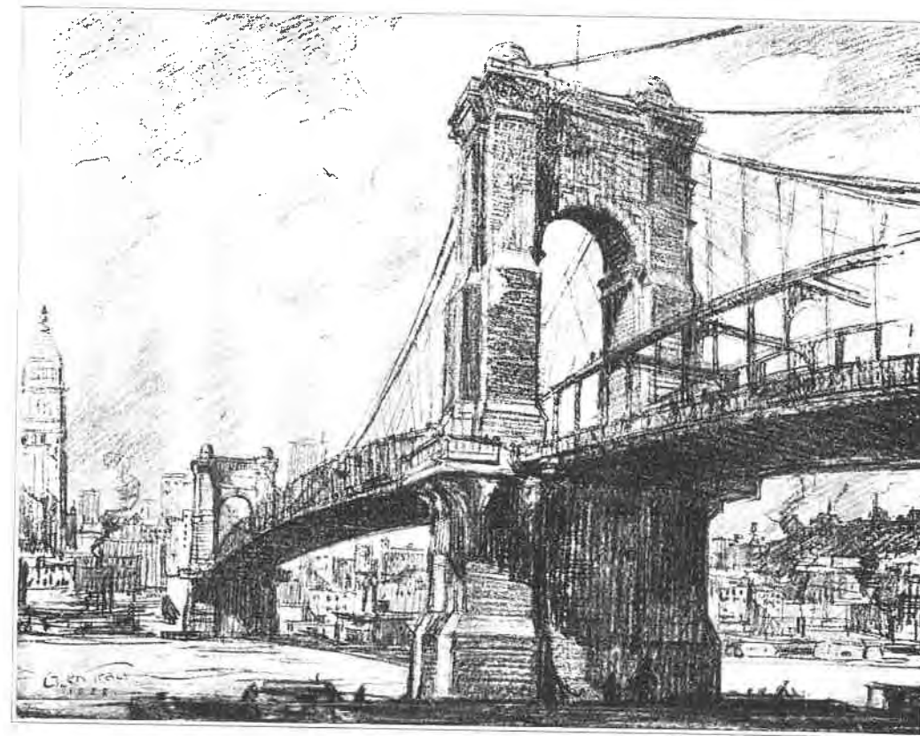
THE OHIO SUSPENSION BRIDGE (Courtesy of Glen Tracy) A worthy approach to the city
