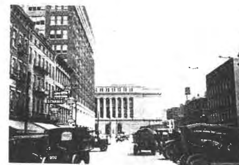
COURT STREET TOWARD COURT HOUSE AFTER WIDENING One half of facade visible
