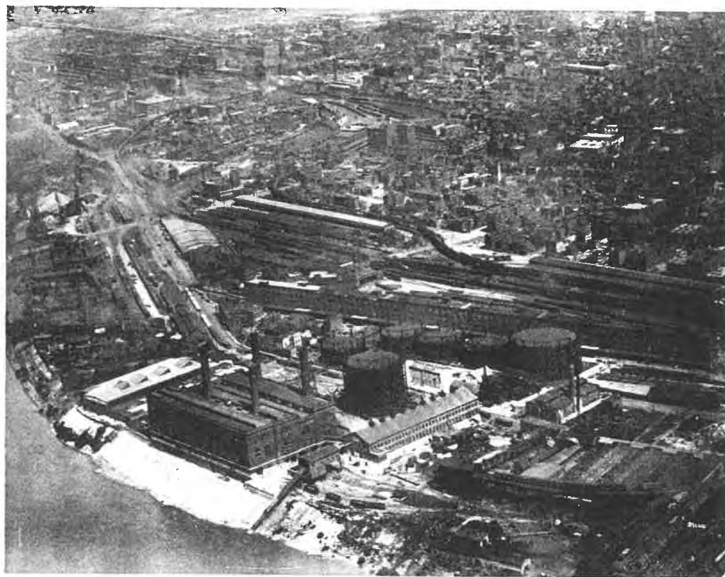
THE "BASIN" FROM THE SOUTHEAST Aeroplane view of railway tracks and freight station network
