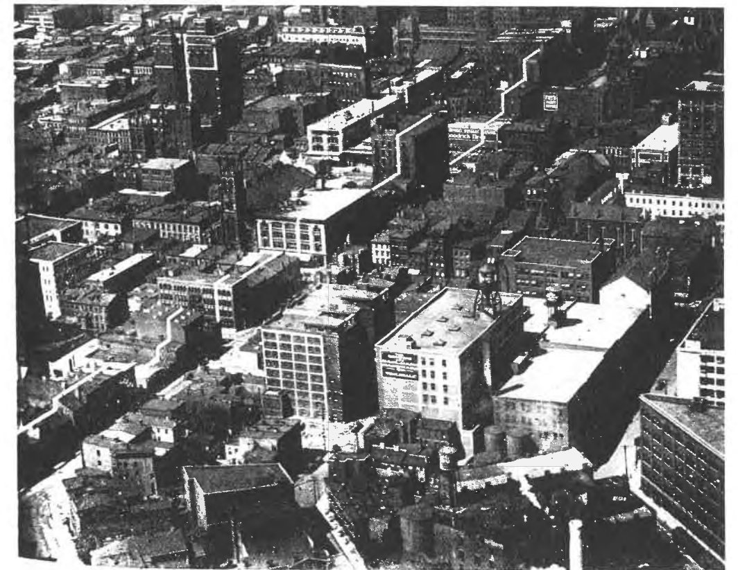
FIFTH STREET EAST Aeroplane view of Fifth Street widening
