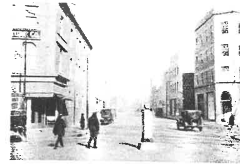
BANK STREET, NORFOLK, VA. Street recently widened twenty feet on the right side, by property owners agreeing to give land, provided the city would pay the cost of setting back the facades.
