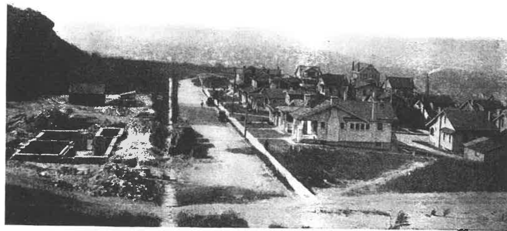
CLEMMER AVENUE, WEST OF HUGHES HIGH SCHOOL Foundations for a macaroni factory in a home district caught by "Zoning".
