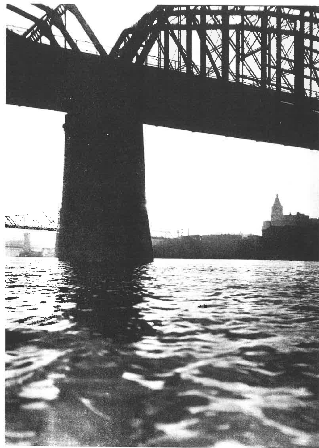
CINCINNATI BRIDGES The city's arteries to the South
