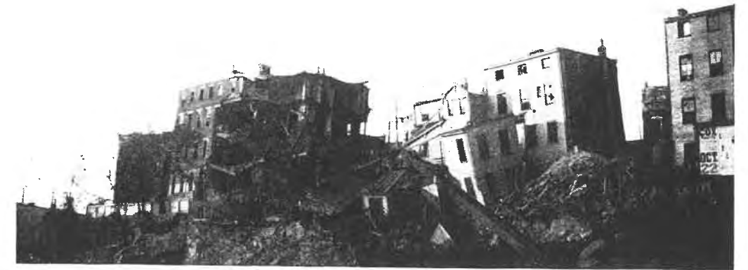
BUILDING COLLAPSING AS THE SIDE HILL SLIPS The steep side hills are often treacherous for buildings
