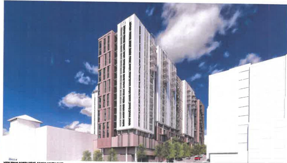
VIEW FROM NORTH-WEST FACING SOUTH-EAST
