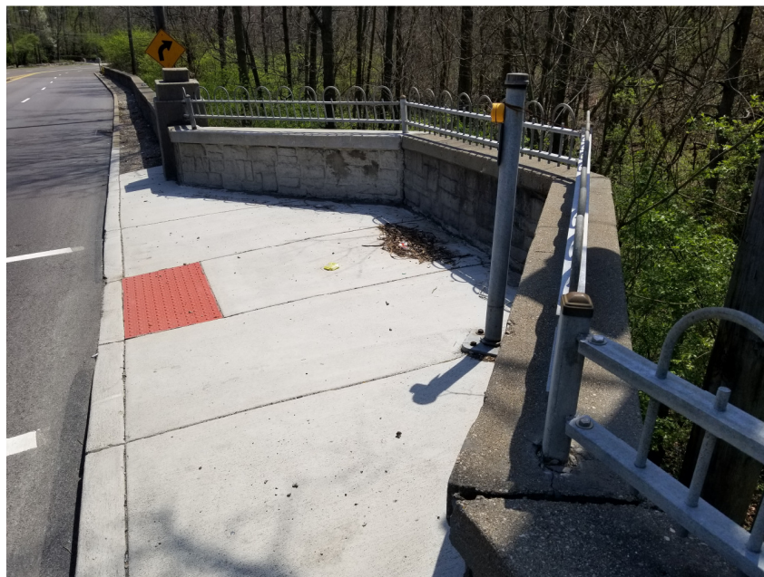
Repaired bus stop opposite Tranquility Lane.
