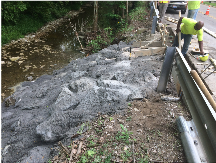
Grouted Rip-Rap at Camargo Road
