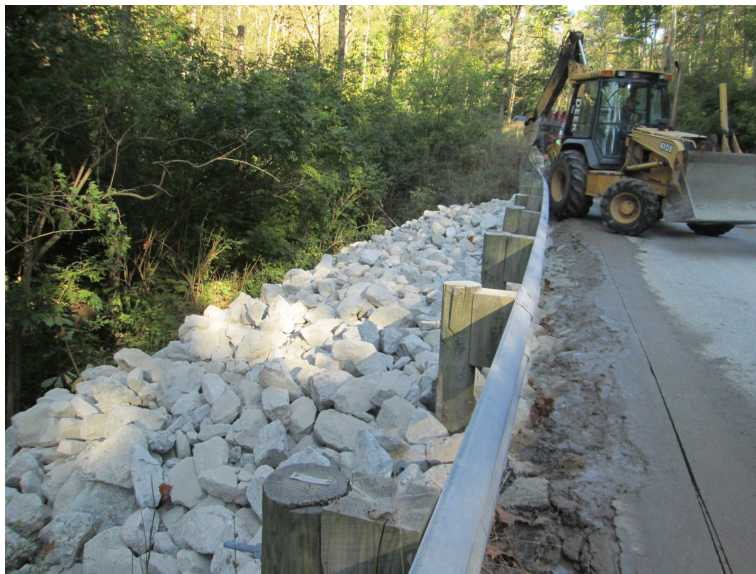
Rip-Rap placed on Kirby Avenue.
