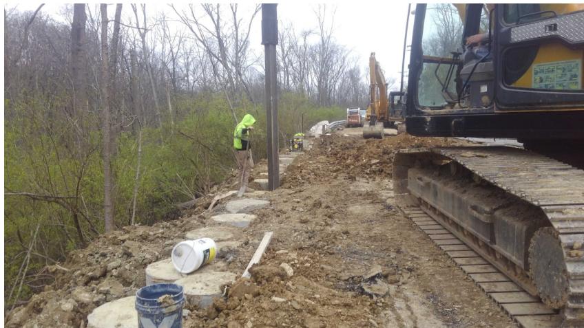
Drilling Piers on Kirby Avenue
