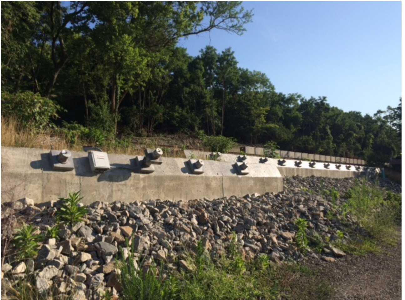
East end of Area 1 Retaining Wall
