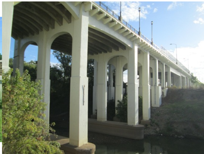
Eighth St. Viaduct
