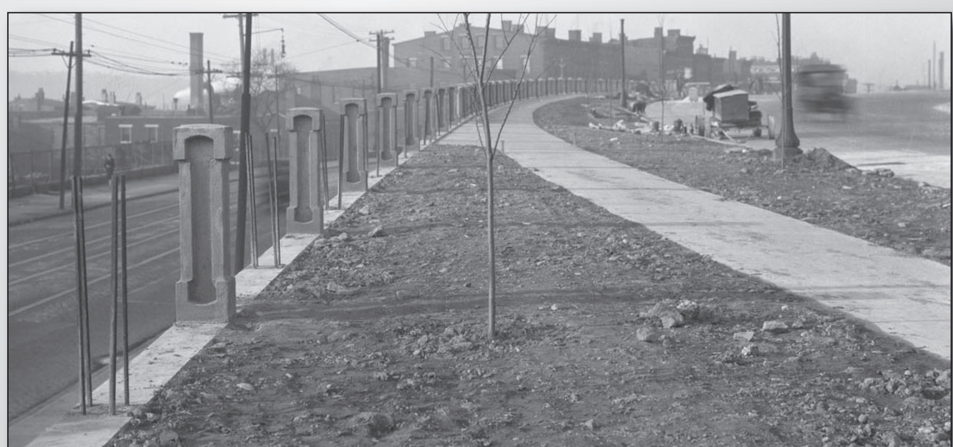
Railing construction along Central Parkway north of Brighton
