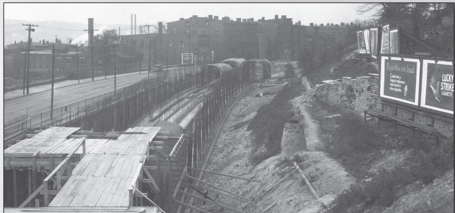
Central Parkway subway tunnels north of Brighton
