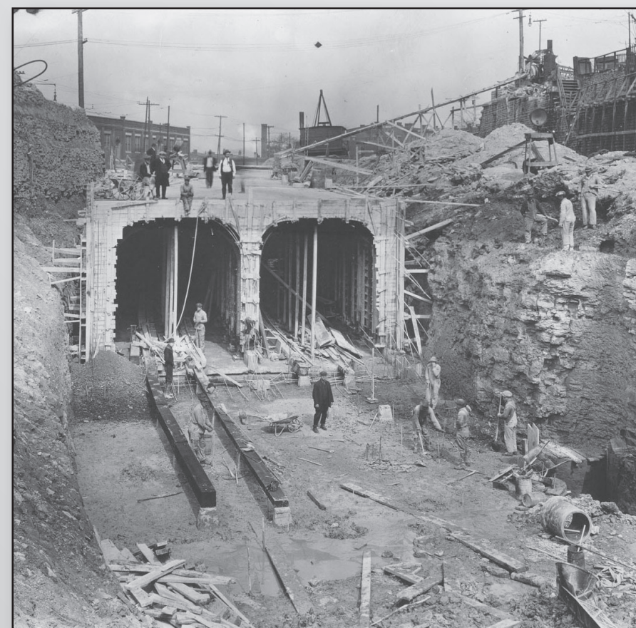
Construction of subway tunnels at Brighton
