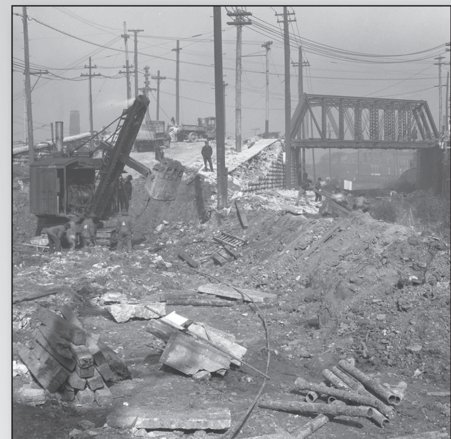
Tearing down Brighton Bridge and clearing canal
