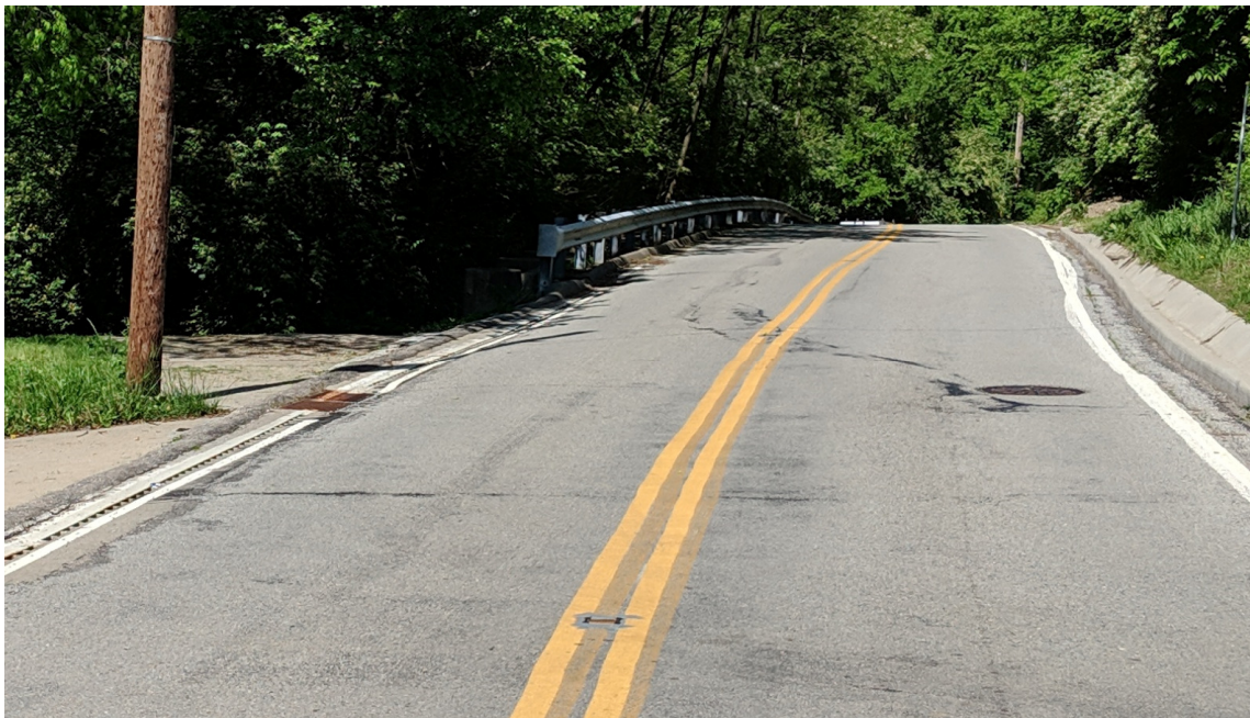
4291-4261 Hillside Avenue (Area 1)
