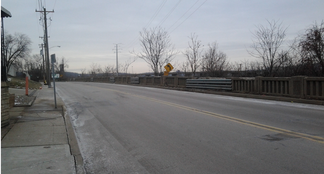
Sections of concrete railing replaced with guardrail sections bolted to pilasters on Cummins Street.
