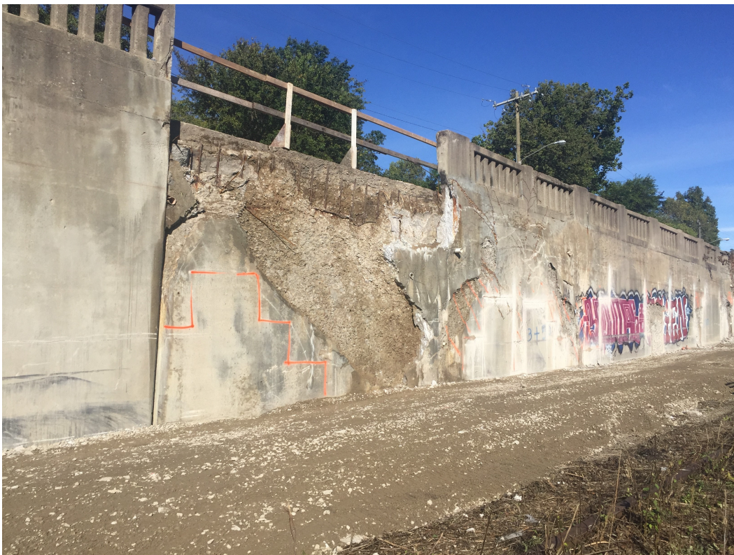
Retaining wall panel after chipping and prior to patching.
