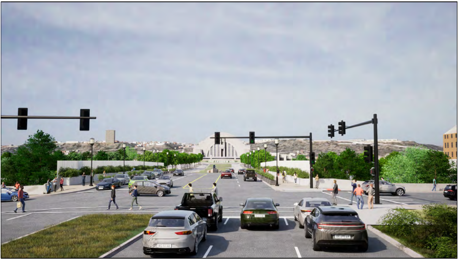
This view shows what the new, two-way bridge on Ezzard Charles Drive will look like. Notice the wide shared use path on the right and the sidewalk on the left. Also notice the planters, screenwall, and decorative lighting on the bridge. The bridge lights and traffic signal supports will be black and meet City aesthetic standards.
