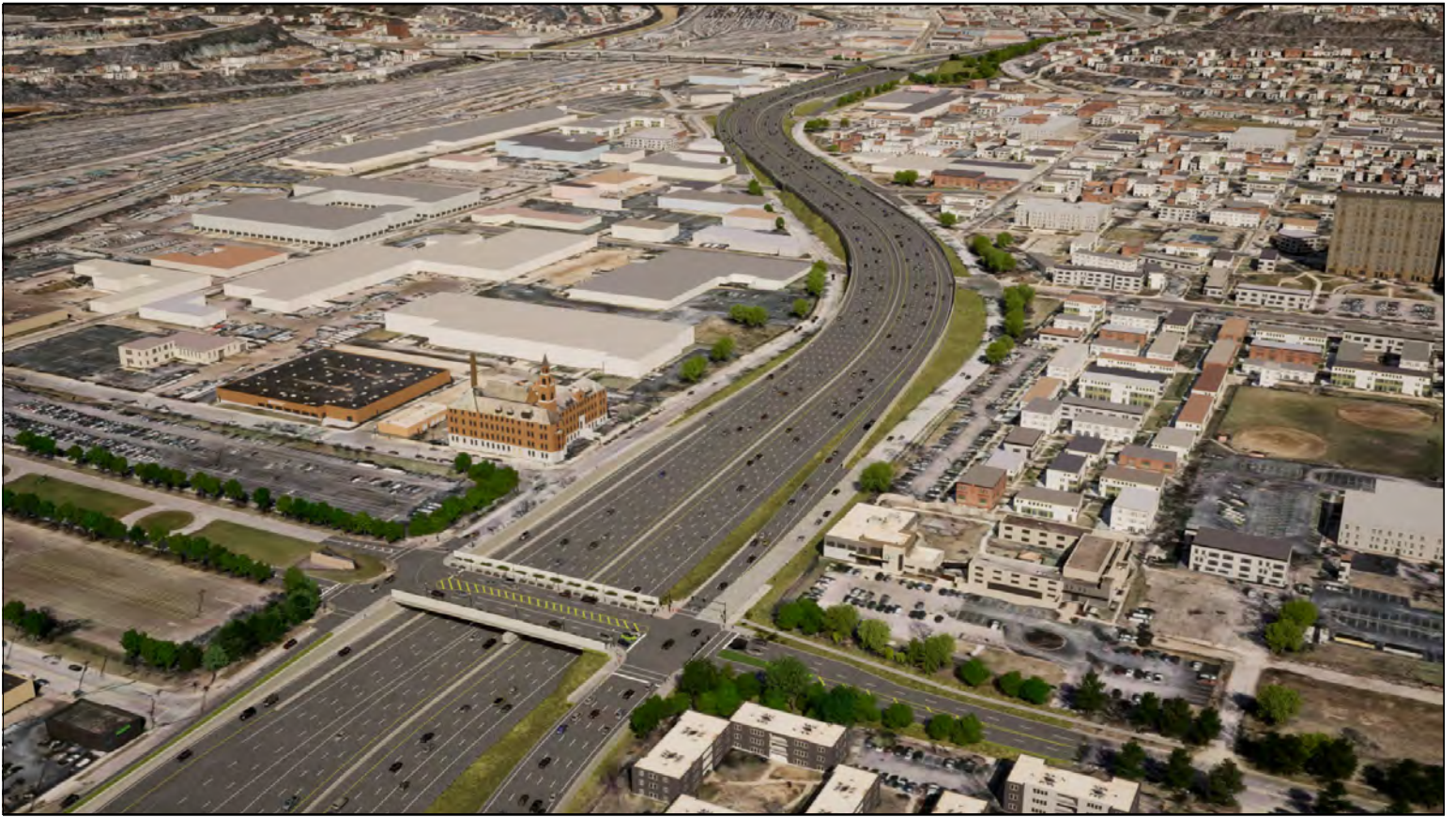
This view shows what the finished project will look like from Ezzard Charles Drive looking north toward Camp Washington. Notice the ashlar stone treatments on the retaining walls.
