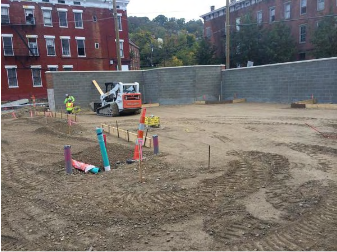
Photo 6: Preparing the sub-base for MOF Concrete Paving
