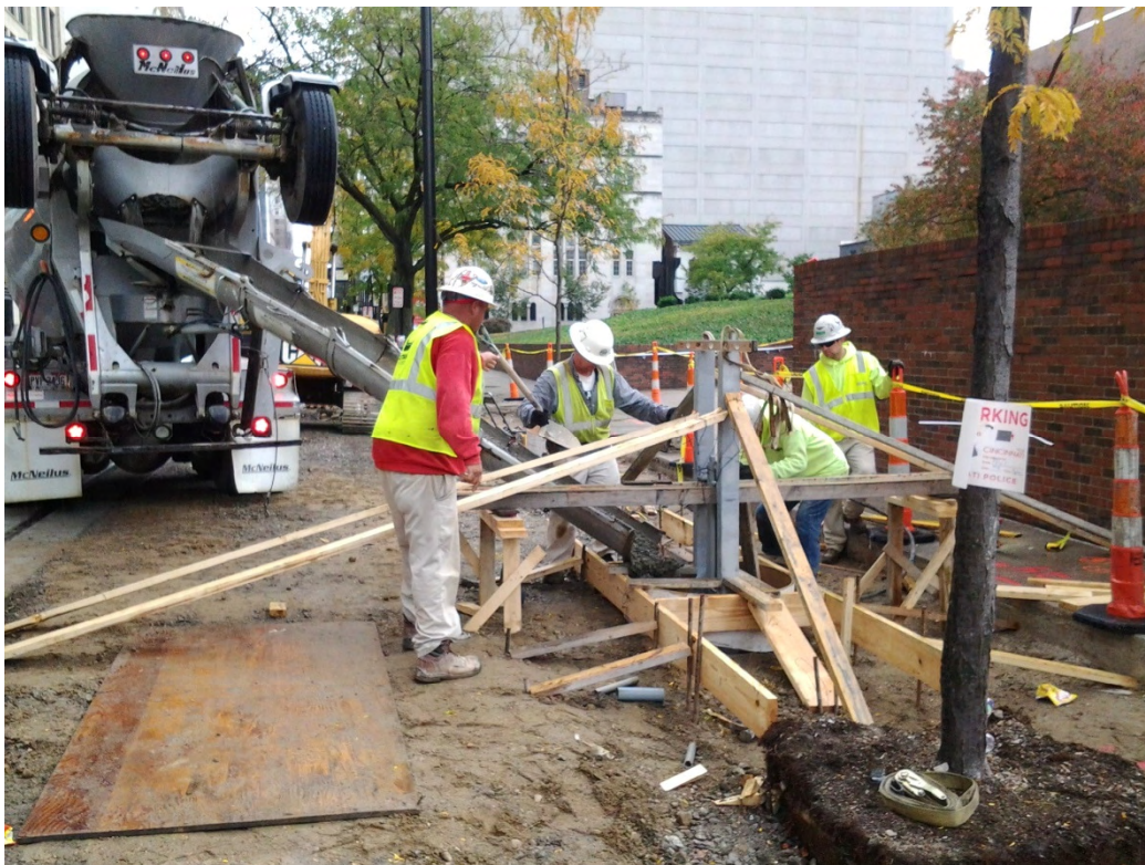
Photo 13: Installing Stop # 15 shelter foundation and support
