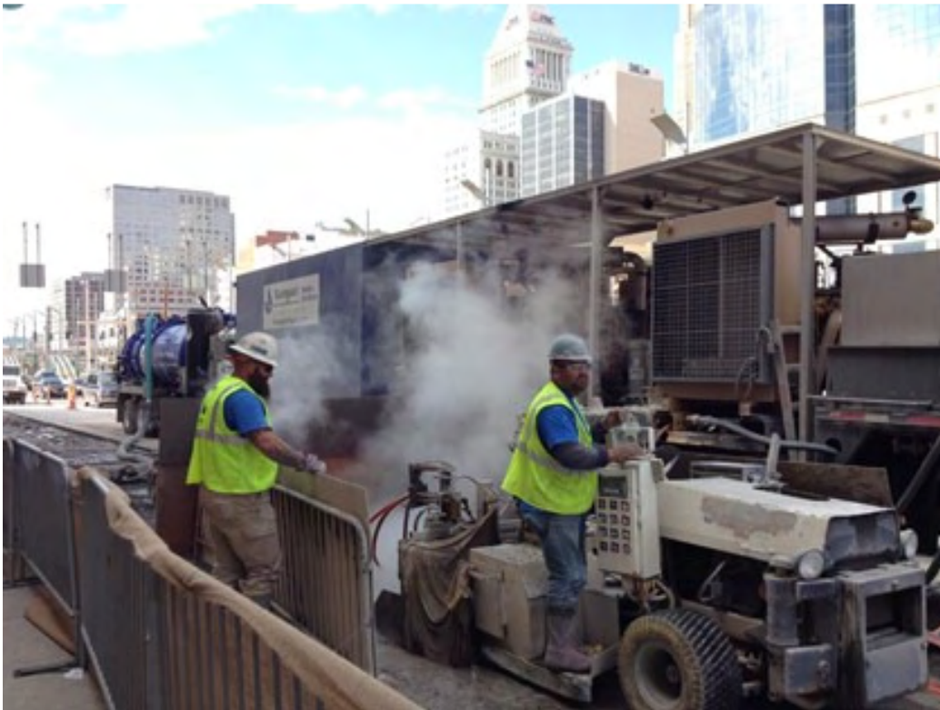
Photo 3: Hydrodemolition on 2 nd street
