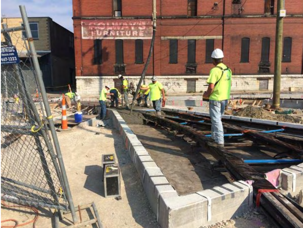
Photo 2: Henry St. tub for turnout to MOF, October 2 nd , 2014
