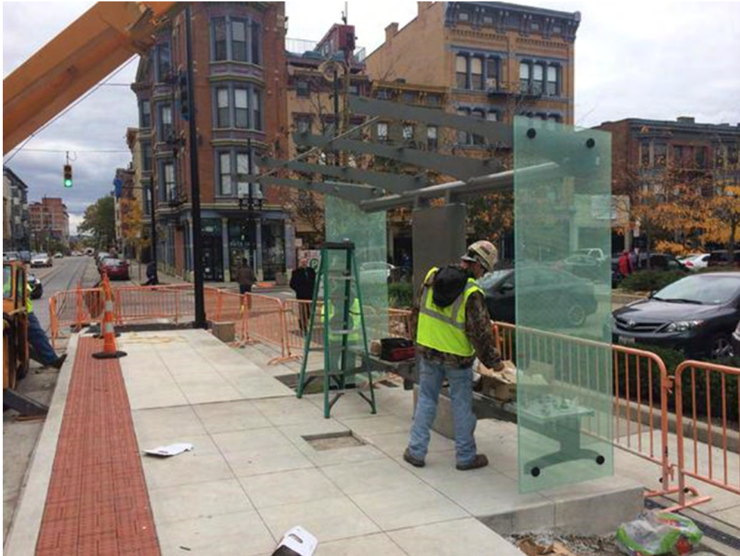
Photo 12: Installing the shelter at Stop #6, 12th St. and Vine St.
