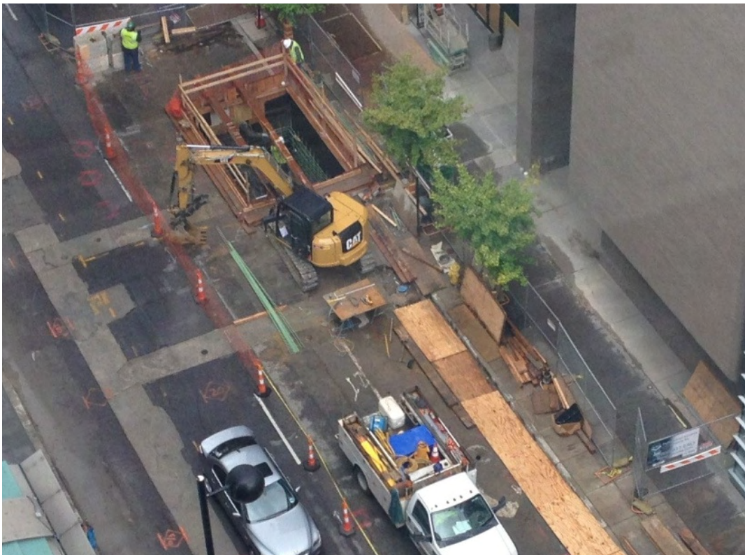
Photo 24: Duke electrical vault reconstruction
