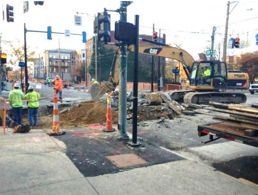
Photo7: Removing Pavement Race St. and Findlay St. during the intersection closure
