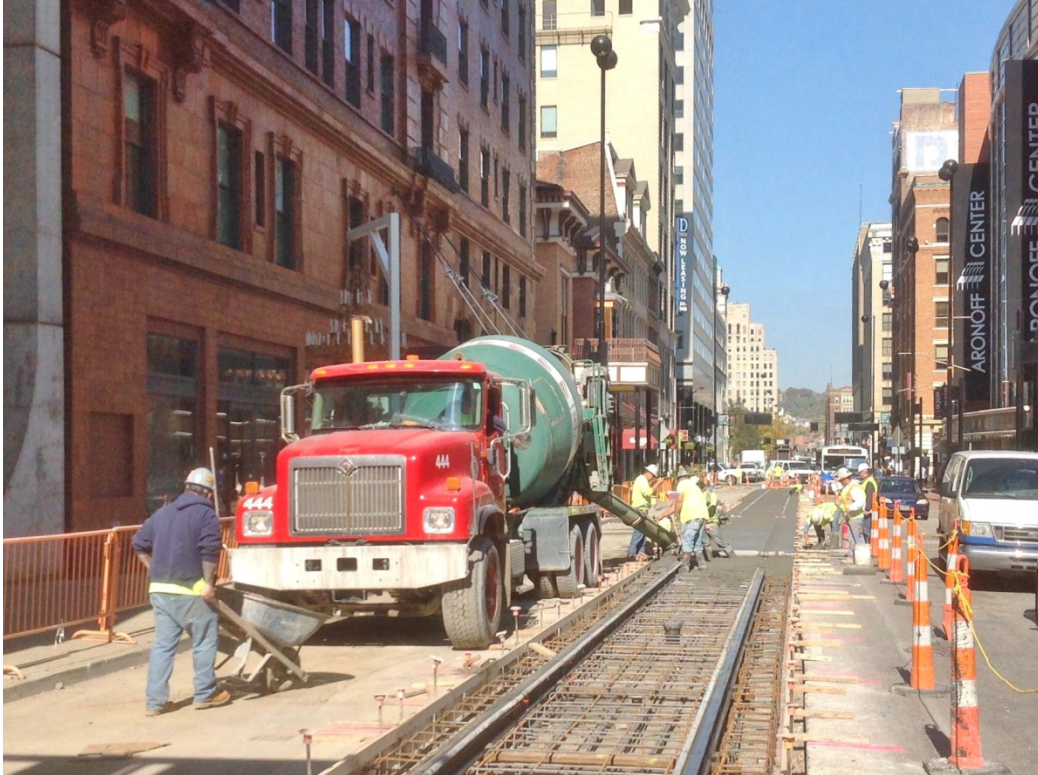
Photo 10: Trackslab concrete on Walnut St, 6th St. to 7th St.
