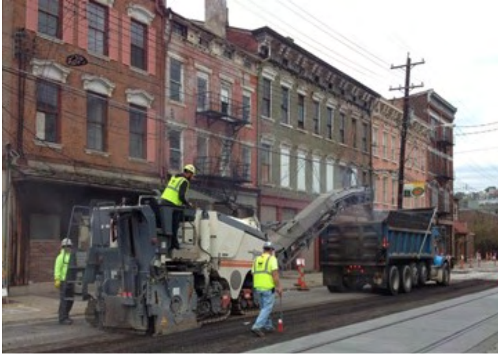
Photo 4: Milling Asphalt on Elm St.
