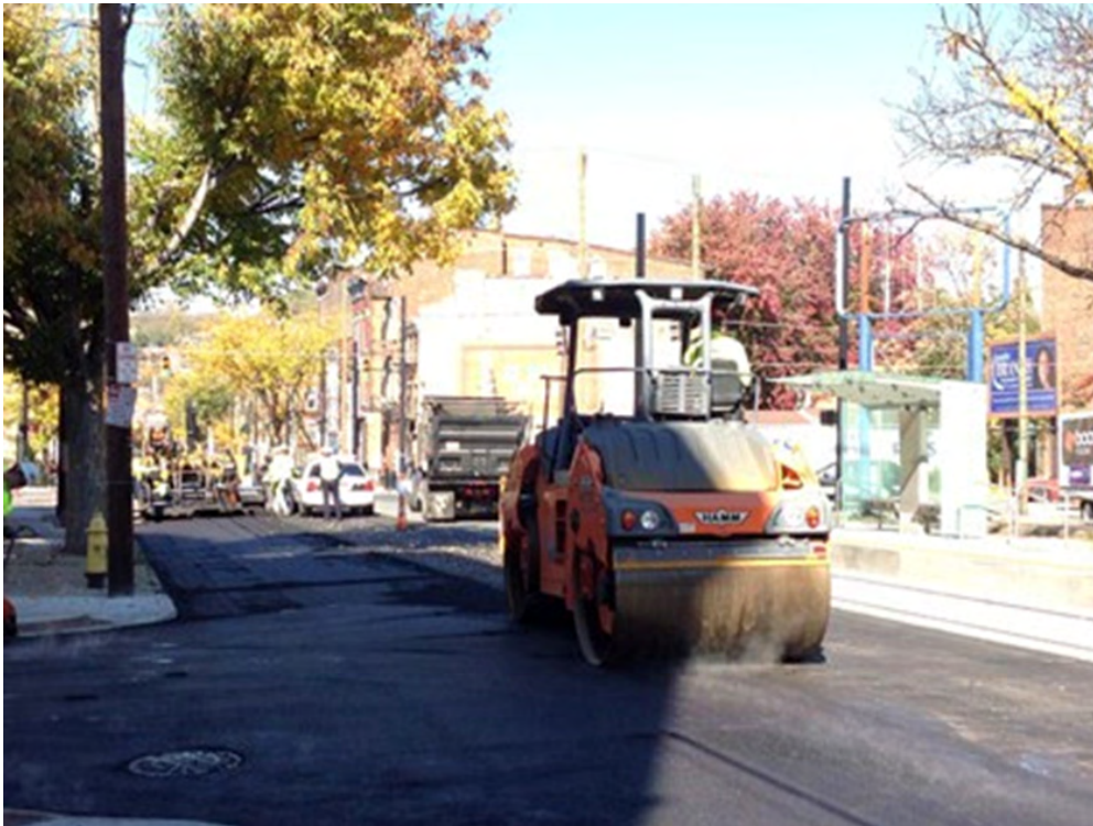
Photo 5: Paving Elm St. near Liberty St.
