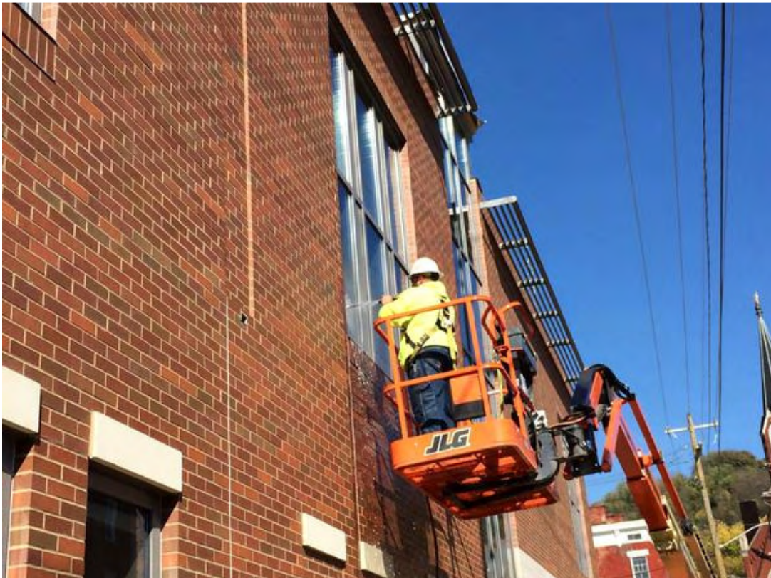
Photo 18: Water testing windows at the MOF
