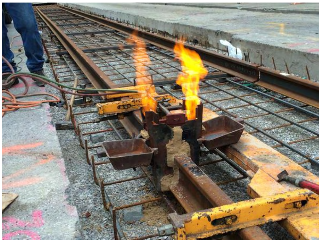
Photo 9: Thermite welding, October 9 th , 2014
