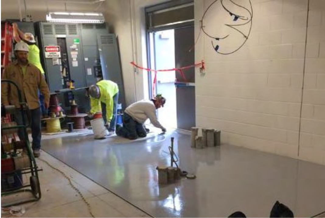
Photo 17: Epoxy floor treatment at the MOF
