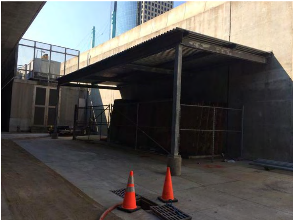
Photo 20: TPSS#1 location prior to demolition of flood gate storage area
