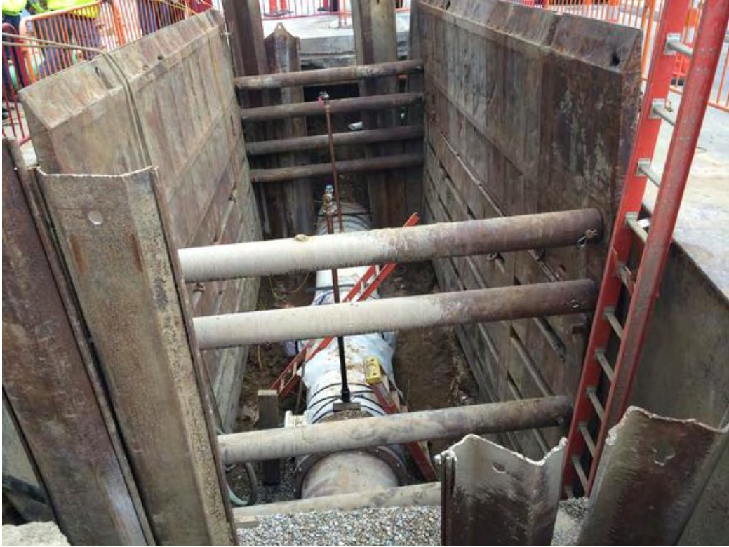
Photo 19: GCWW valve replacement at Central Parkway & Main
