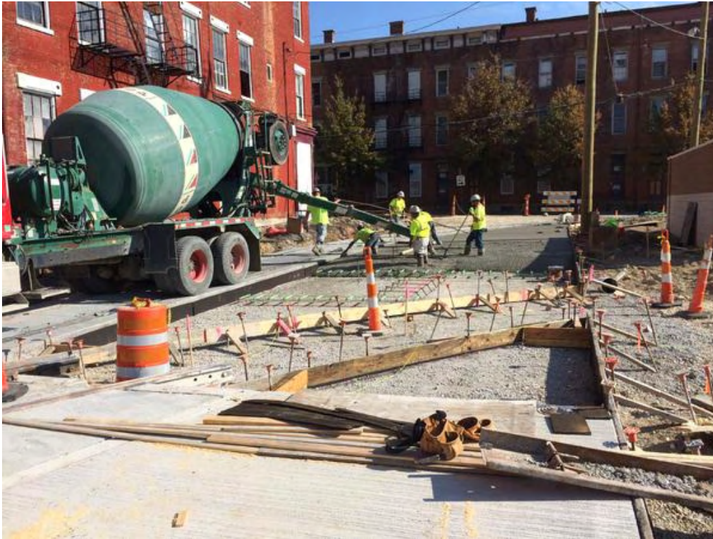
Photo 8: Replacing Pavement Henry St. & Race St. October 27 th , 2014
