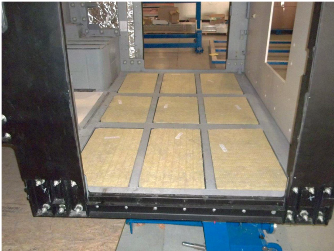
Photo 28: Insulation installed in floor panel
